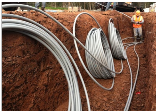
Figure B.6 Horizontal Geothermal Application
