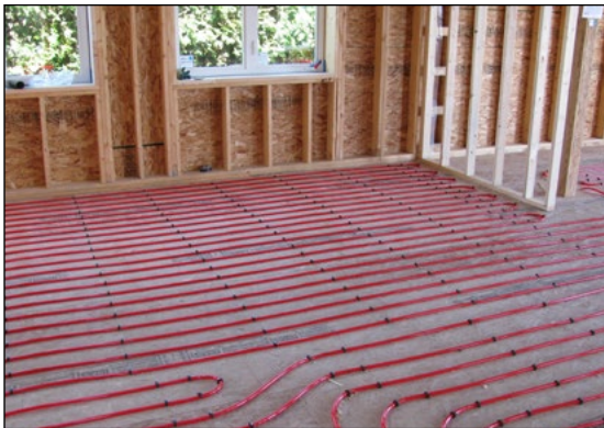
Figure B.1 Radiant Floor Heating Tubing in a Residential Application
